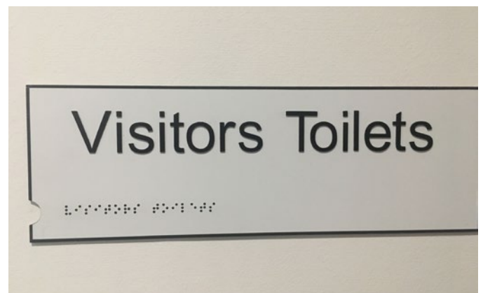
■ A detail of the tactile sign board used to locate braille messages
