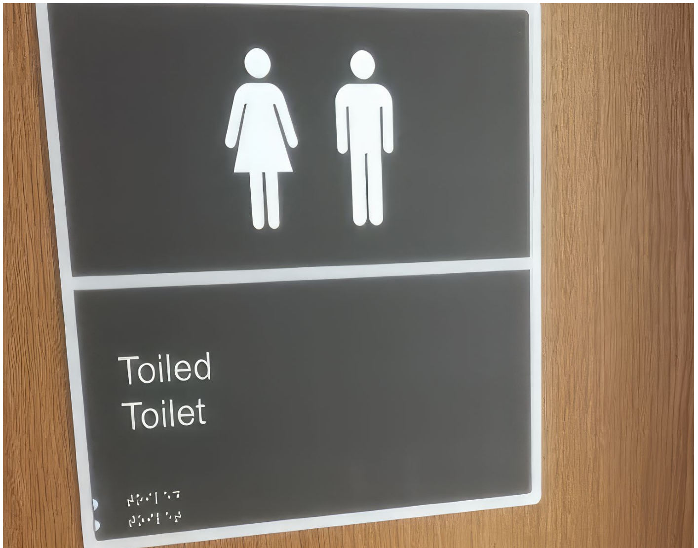
■ Toilet signage, contrasted sign at eye level with tactile images, words and braille.
