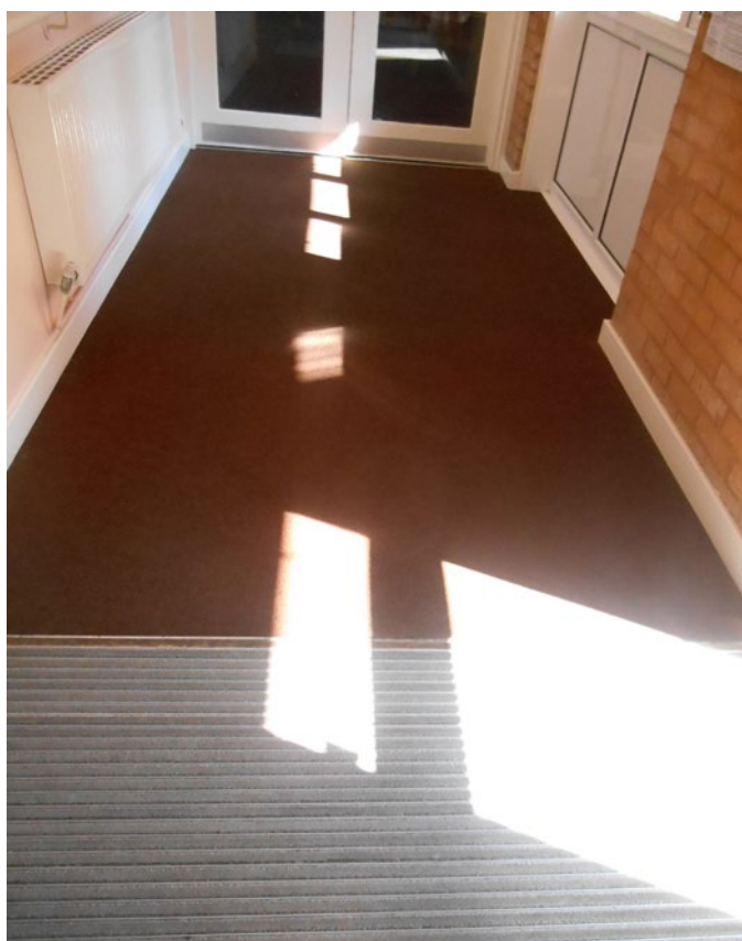
■ Overhead lighting and no window protection causes areas of glare on the ceiling and floor
